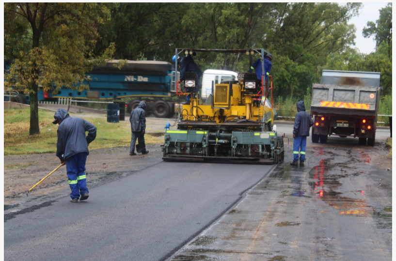
Workers Place Romix RoadSafe on Road in Rainy Conditions, Senekal, South Africa.
