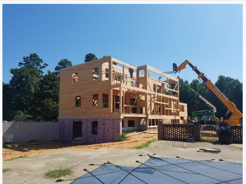
Solar Meridian in Charlotte NC under construction
