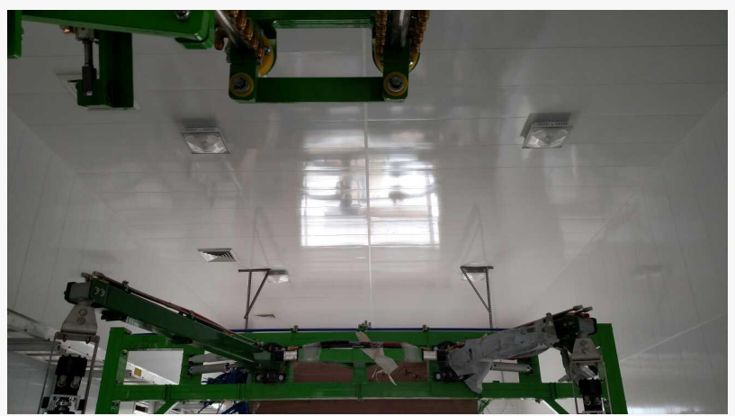
UtiLite Ceiling Panels in a Carwash.
