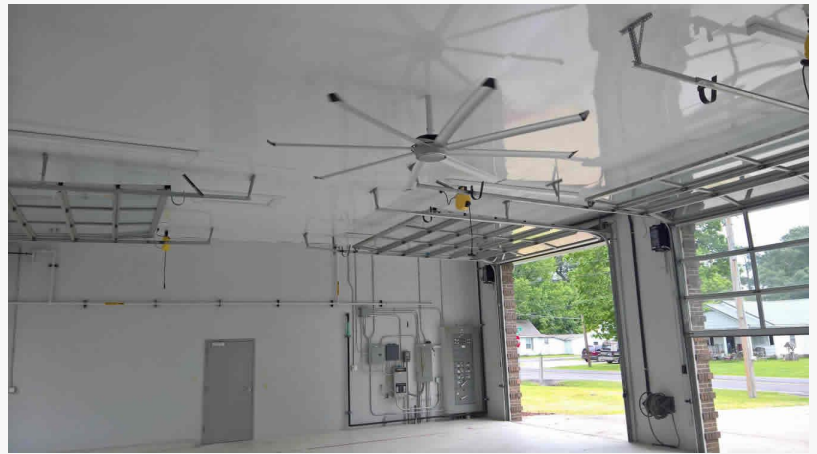
UtiLite Ceiling Panels in a Fire Station.
