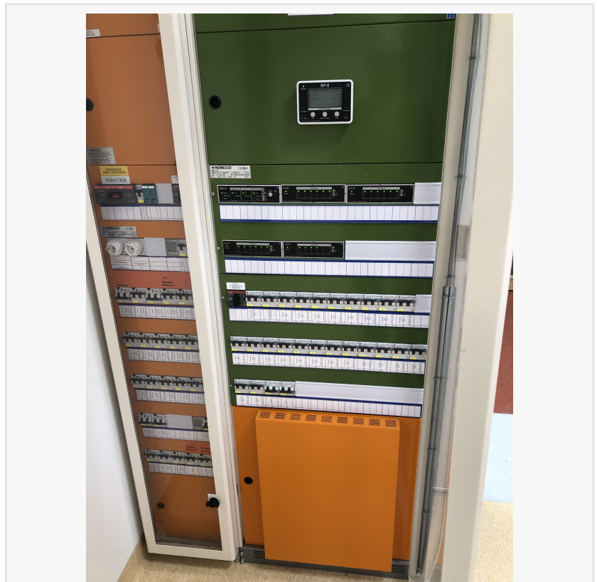
MEV-8 Insulation Monitoring System in an IPS rack
