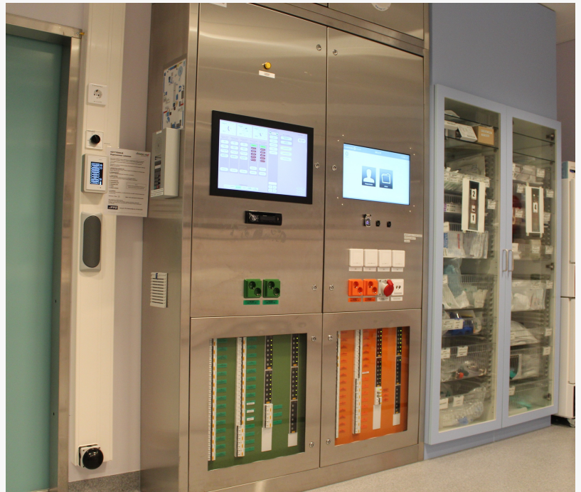
MEV-8 Insulation Monitoring System in the Finnish operating room.
