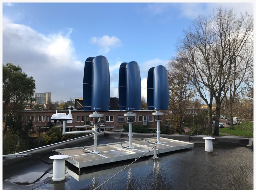
Three installed small size Wind Tulips
