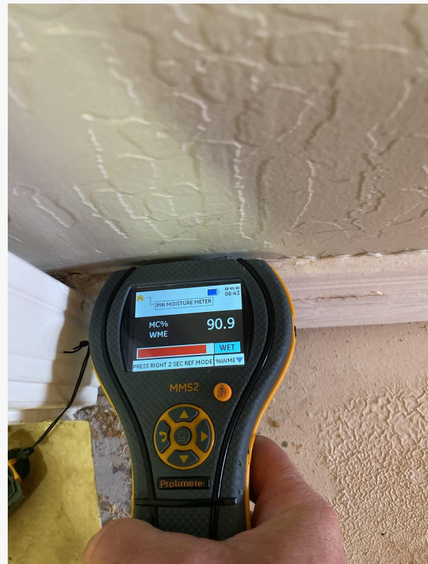
Finding water hidden in the walls.
