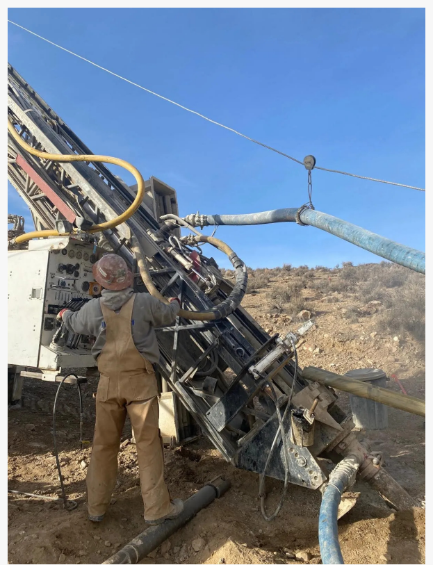
Independence drilling operations
