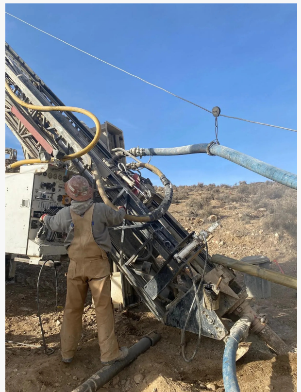
Independence drilling operations
