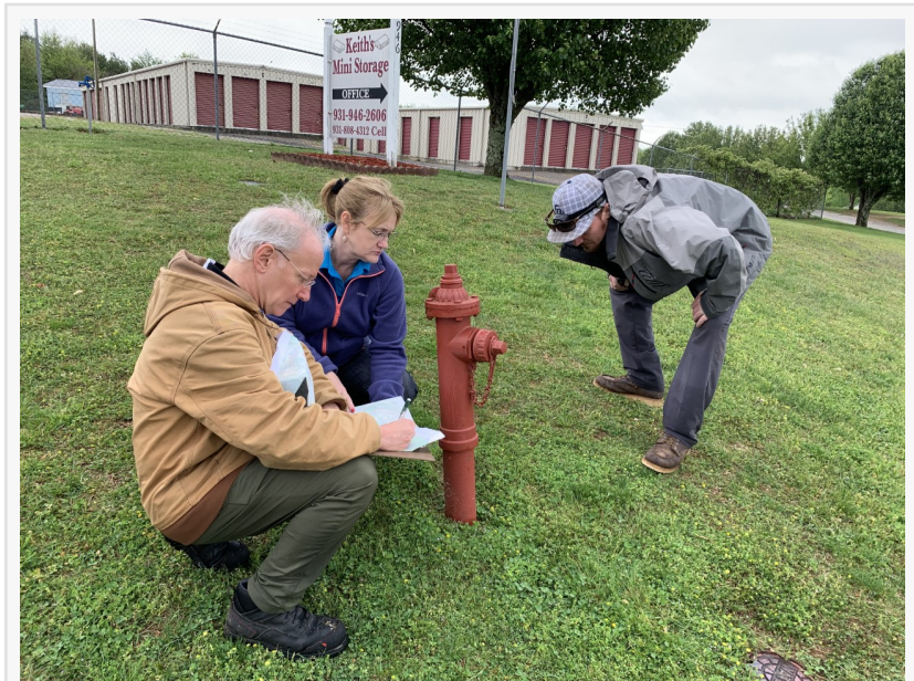
Paul Pasko, Electro Scan, Zeda Hillis, J.C. Haley, and Douglas Cole, Spencer Utility, evaluating insertion points for entry into the City's potable water network.
