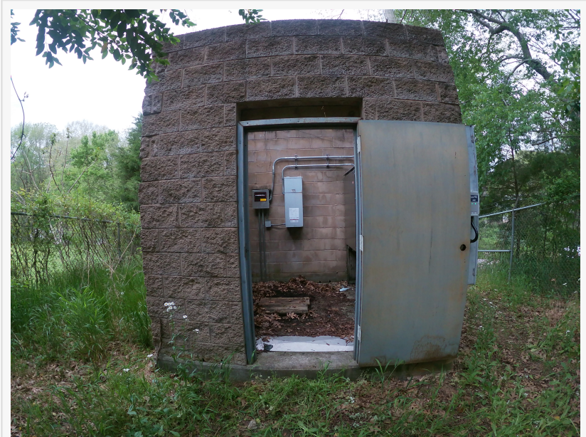
Raw water line's pump house at the edge of the Caney Fork River.
