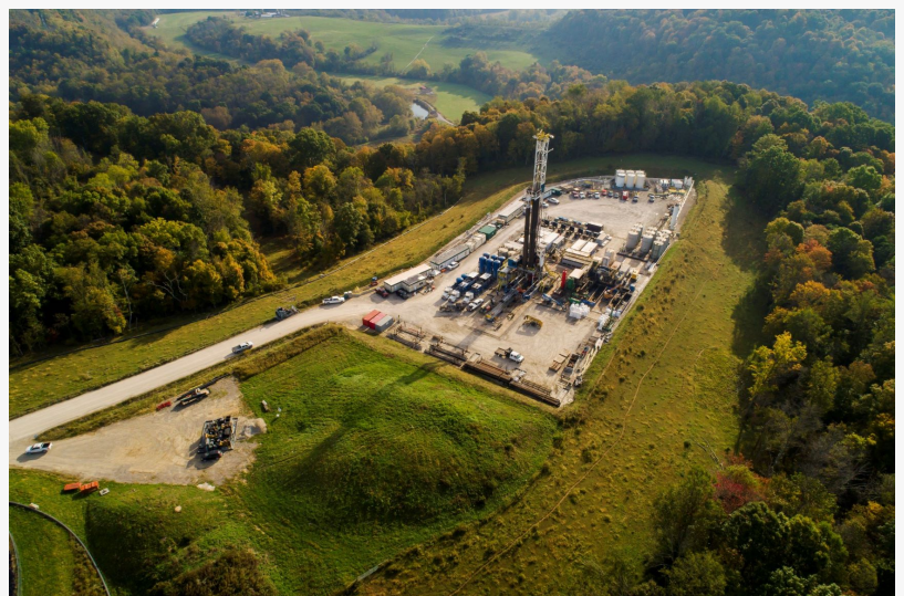
Ohio County, WV Drilling Rig
