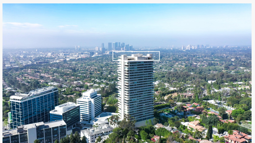
Sierra Towers Penthouse, 9255 Doheny Road #PH1 & 2, West Hollywood, CA
