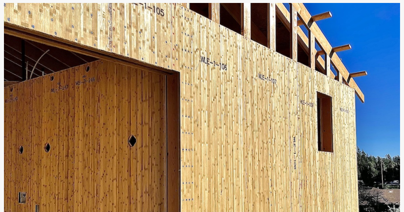
BamCore Gen 3 stud-less framing solution reduces over 80% of studs, headers and posts.
