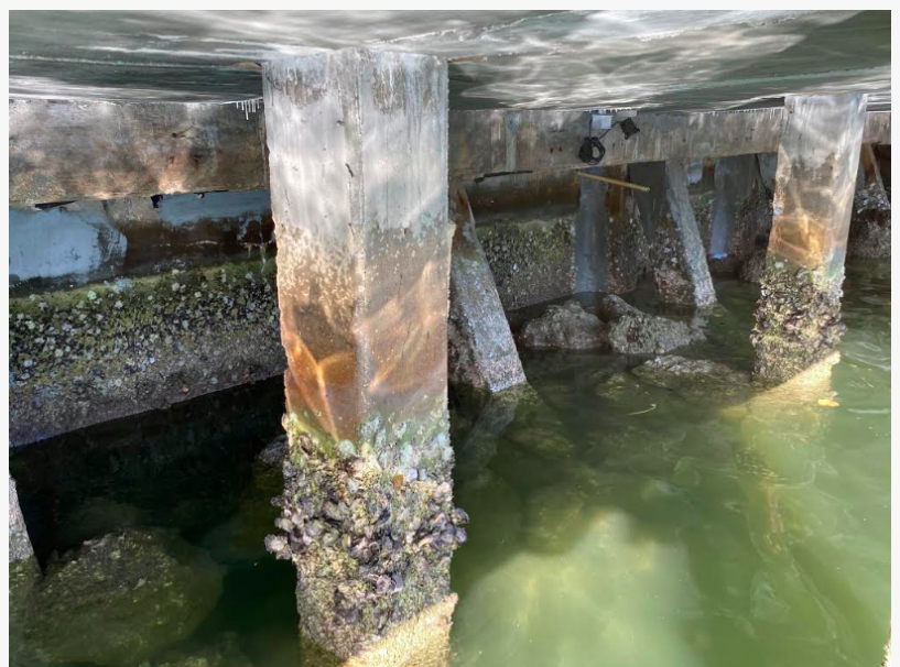
Seawall Repair done in Fort Lauderdale FL
