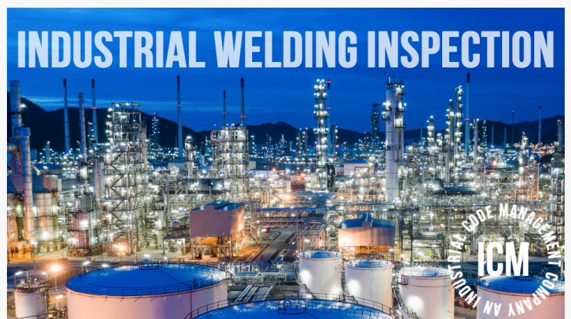
Industrial and Commercial Site Quality Control Management Services
