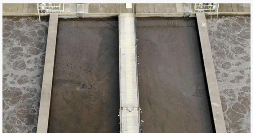
During BioMix-DC's deep cycle, mixing is suspended to allow solids to accumulate.
