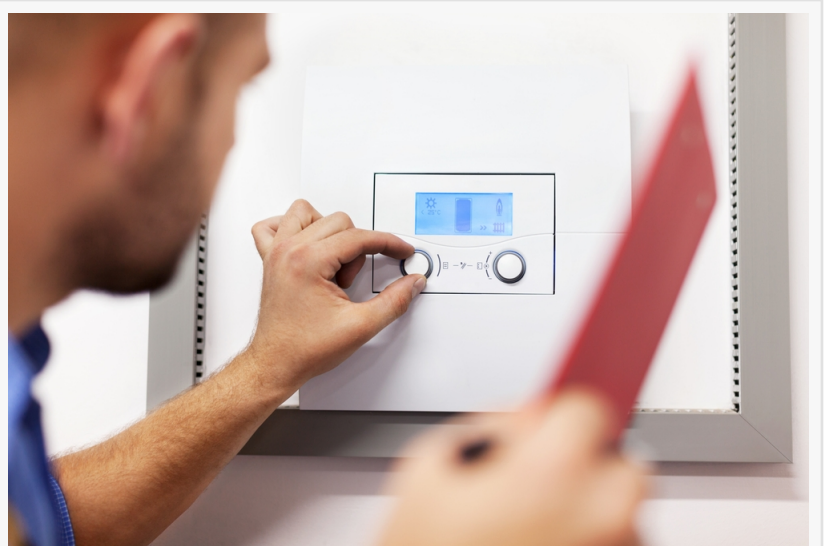
Tankless Water Heater Installation in Tucson
