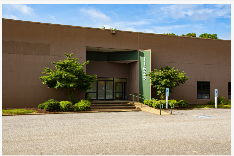
In-Charge Energy's new R&D Facility in Richmond, Va.
