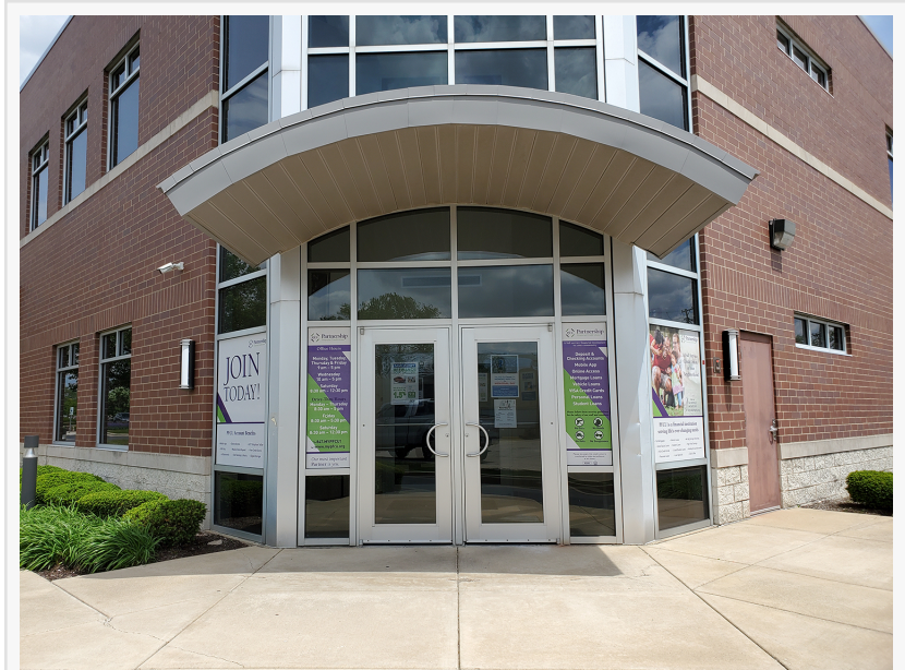
New PFCU location at 2701 N. 25th Ave., Franklin Park, IL.
