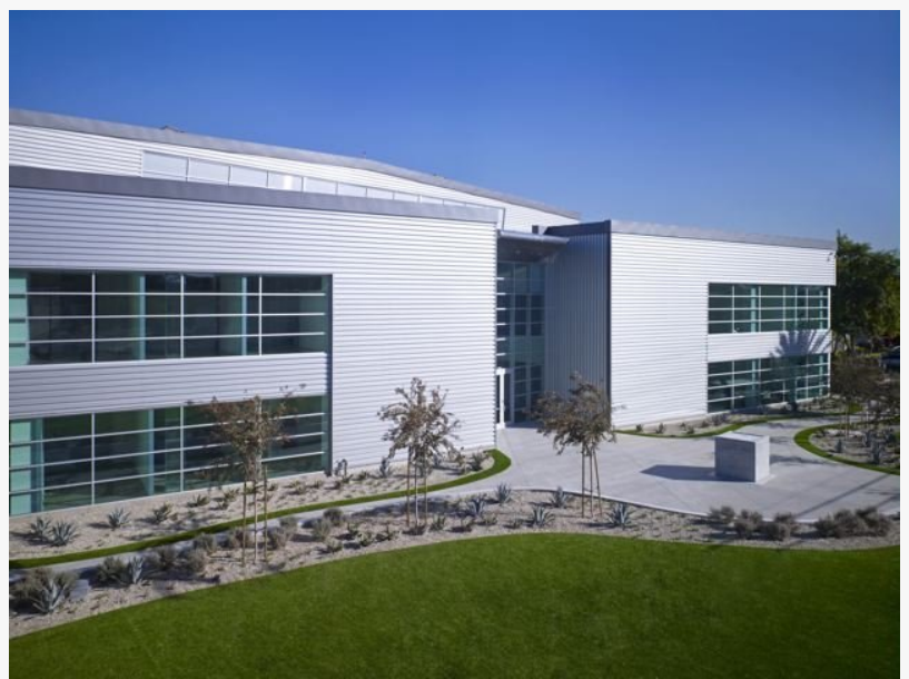
Bob Hope Airport – Hangar 25
