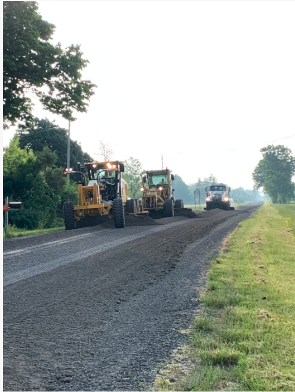
The Flushing road being constructed with Perma-Zyme
