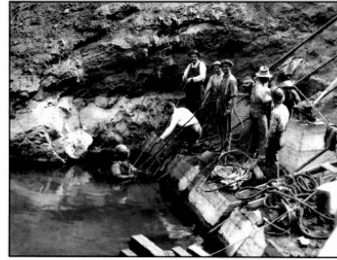
Figure 59. Construction of COPCO No. 1 in 1917 (Photo courtesy of Siskiyou County Museum, Yreka, California, P13668 OS COPCO 2).
