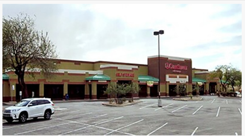
DealPoint Merrill Sells Self-Storage Facility, Chandler, AZ
