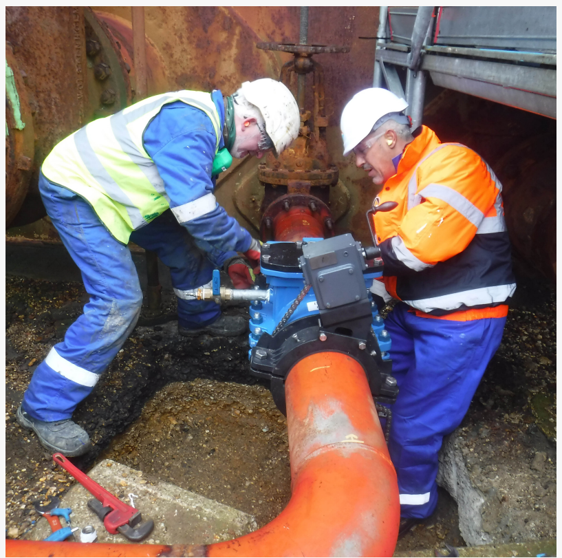
AVT EZ Valve being installed at a UK refinery 2
