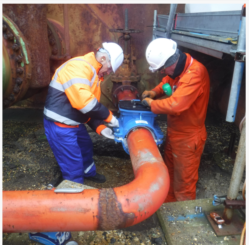
AVT EZ Valve being installed
