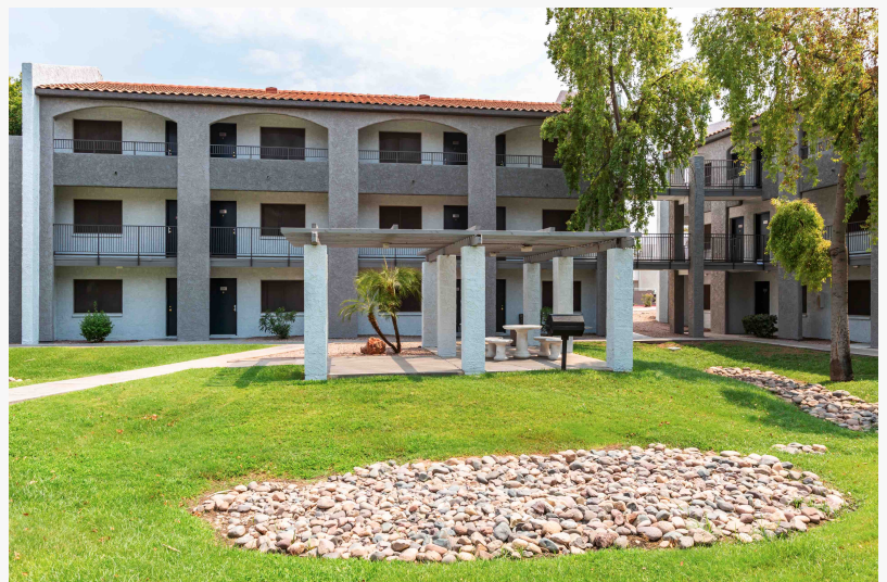
IVilla Garden Apartments, a 214-unit multifamily project in Phoenix
