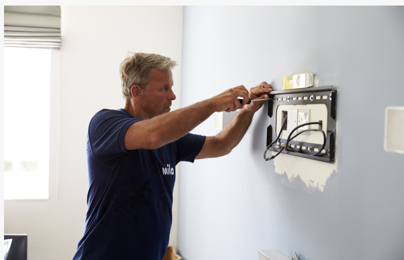
A Mila technician installs a wall mount for a smart TV.
