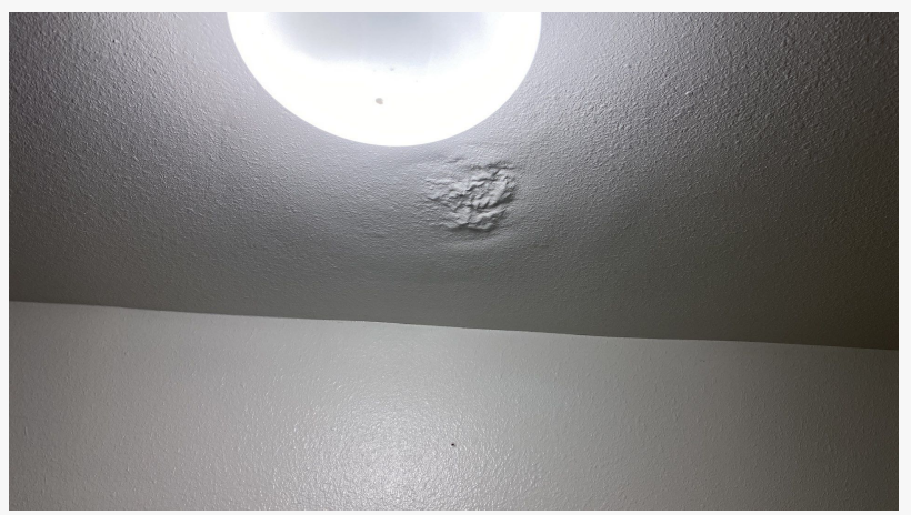
Water Damage in a Kitchen Ceiling.
