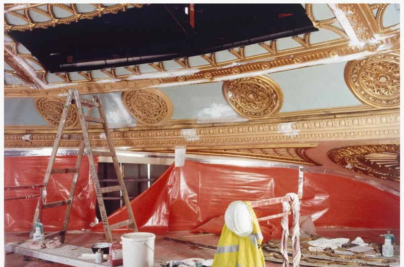
Previous repairs to the fifth floor by a specialist
