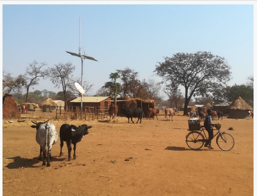
AMN rural mobile network base station in Africa
