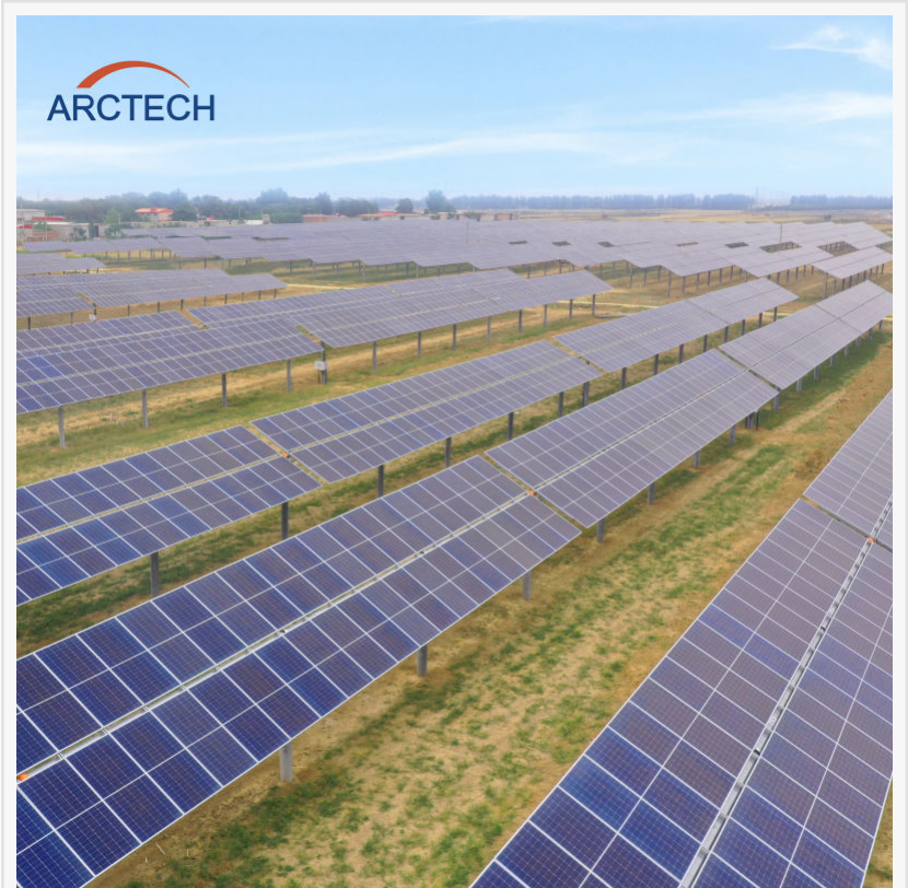
Picture of Arctech's 575MW solar project located in Hebei Province, China
