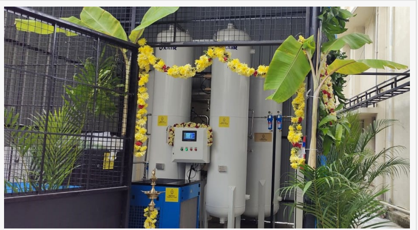
Oxygen Plant at Maharaja Agrasen Hospital in Bangalore
