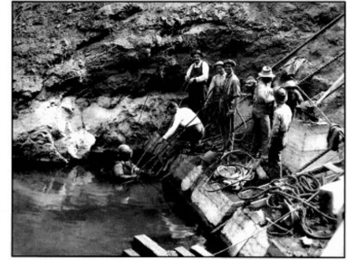
Figure 29. Construction of COPCO No. 1 in 1917 (Photo courtesy of Siskiyou County Museum, Yreka, California, P13668 OS COPCO 2).
