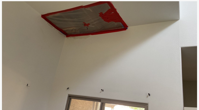
The unit above this client's had a pipe burst and the water leaked through the ceiling.
