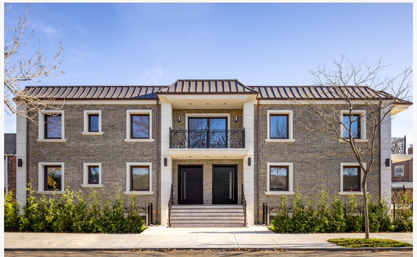
Middle Village is the first precertified passive house in Middle Village, Queens.
