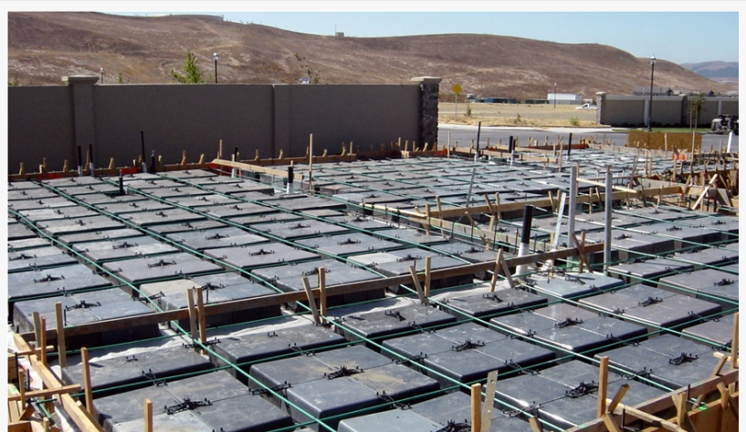
Wafflemat has installed over 30,000,000 SQ Feet of Concrete Foundation with 0 Structural Failures
