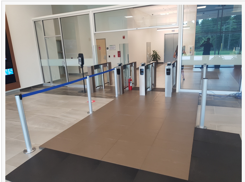
Stepscan Secure Security System installed at the Cyber Center in Fredericton NB, Canada
