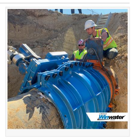
With this configuration, when City engineers need to carry out repairs or maintenance on the towers, they are forced to shut down the entire water system meaning the town has just two hours until all water pressure is lost. The city needed to install a new control point on the system which would enable each tower to be independently isolated allowing the other tower to maintain the city's water supply.
