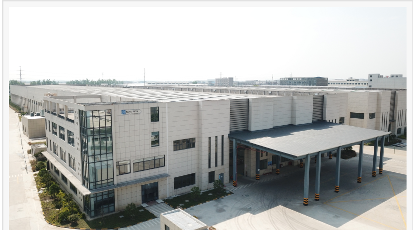
Kautex Pinghu: Future site of Kautex's first compression molding line in China
