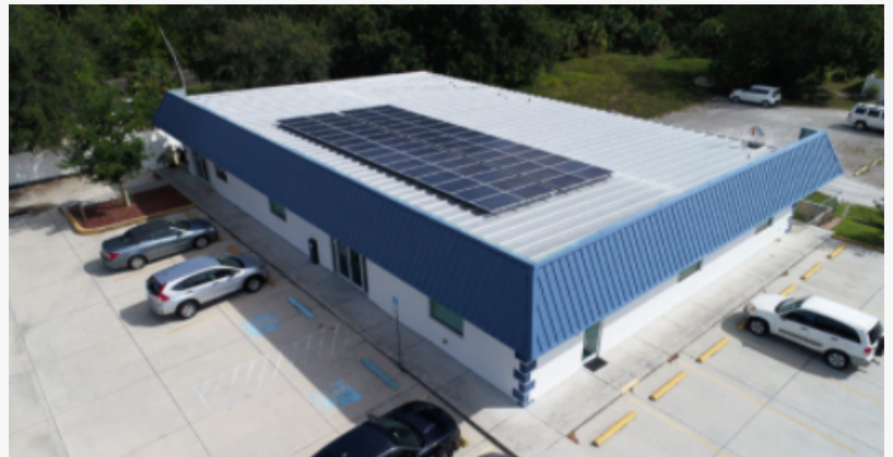
Rooftop Commercial Installation
