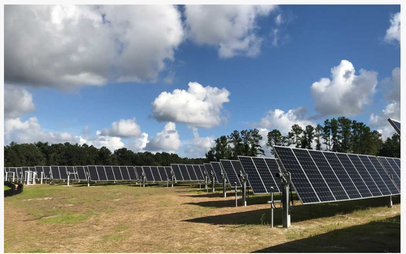
Solar Farm Installation
