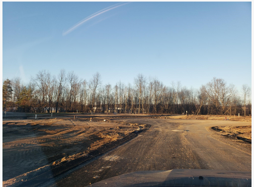
Developing roads for a new manufactured home community expansion
