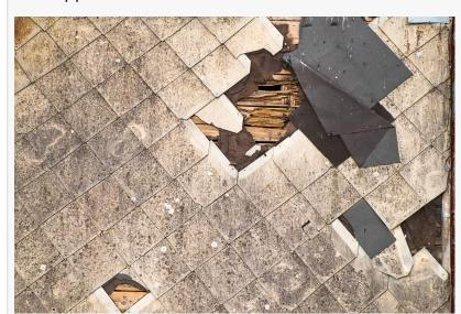
For decades throughout the twentieth century, a mixture of asbestos and cement was used to produce roof shingles.
