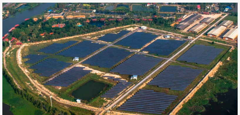
Recent Solar Project
