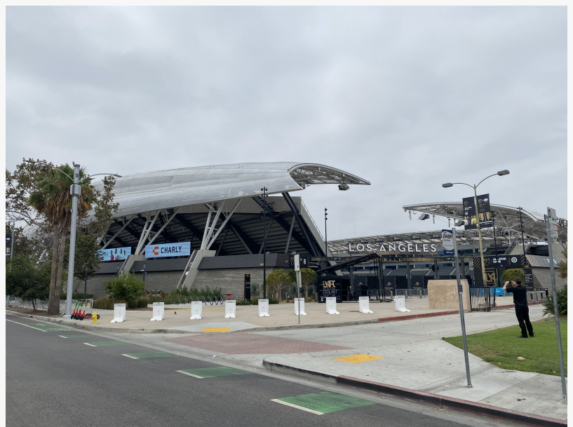
Barriers surrounding Banc of California Stadium
