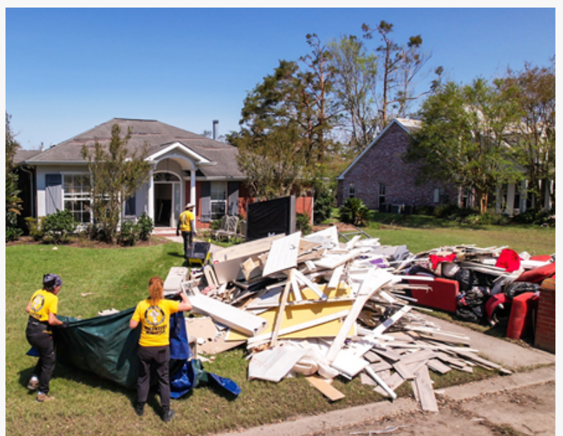
Mucking out a house swamped by five feet of storm water
