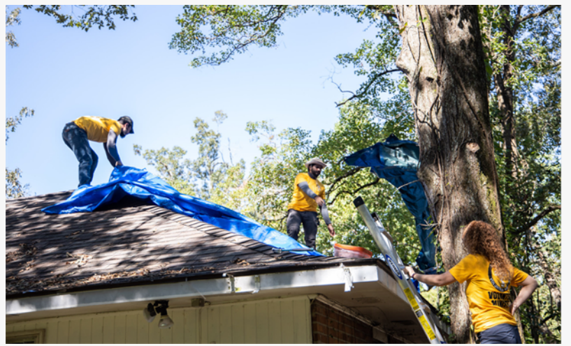
Blue tarping a home to keep future rain out
