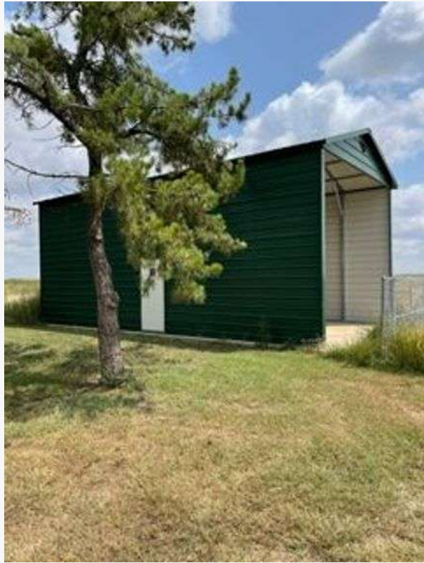
11700 S. Masterson Road, Amarillo, Texas 79118
