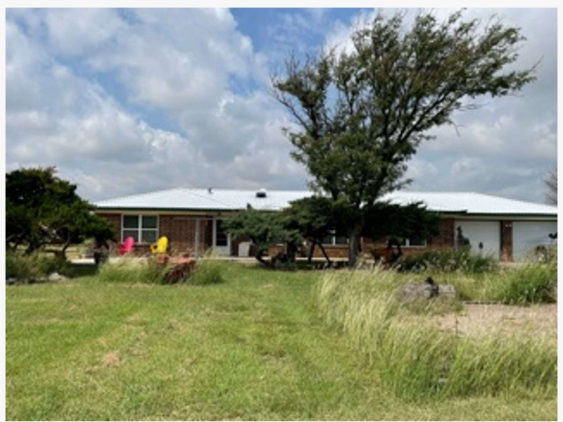
11700 S. Masterson Road, Amarillo, Texas 79118
