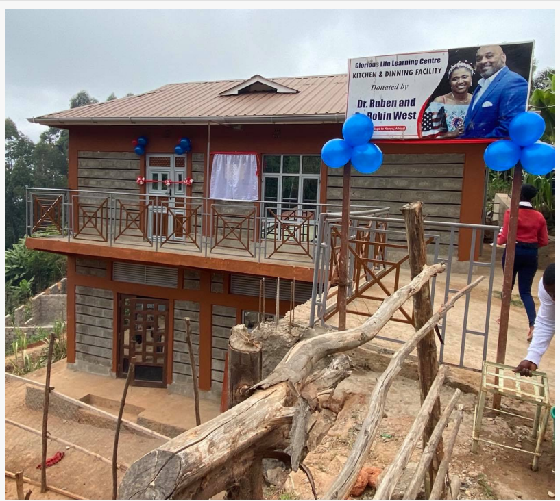
The Rosetta M. West Kitchen & Dining Facility
