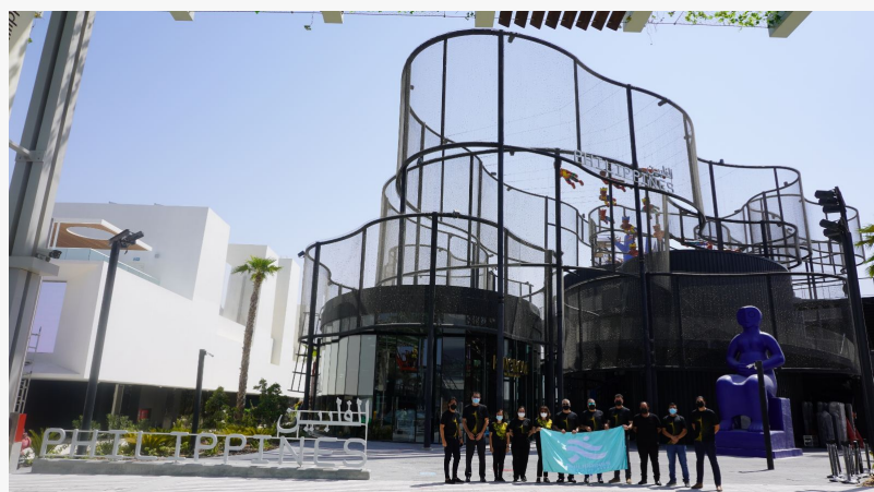
The Philippines pavilion, “Bangkóta” at the Expo 2020 Dubai, with Philippines Expo 2020 Dubai Alternate Commissioner General Rosvi Gaetos (fifth from left), PDTI representatives, and RAQ Contracting Co. LLC senior officials
