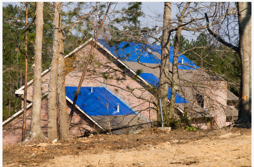
Stopping water damage with tarps
