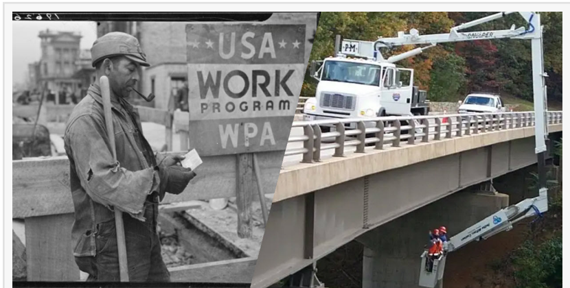
1939 photo by the Works Projects Administration, and 2021 photo by the Federal Highway Administration
