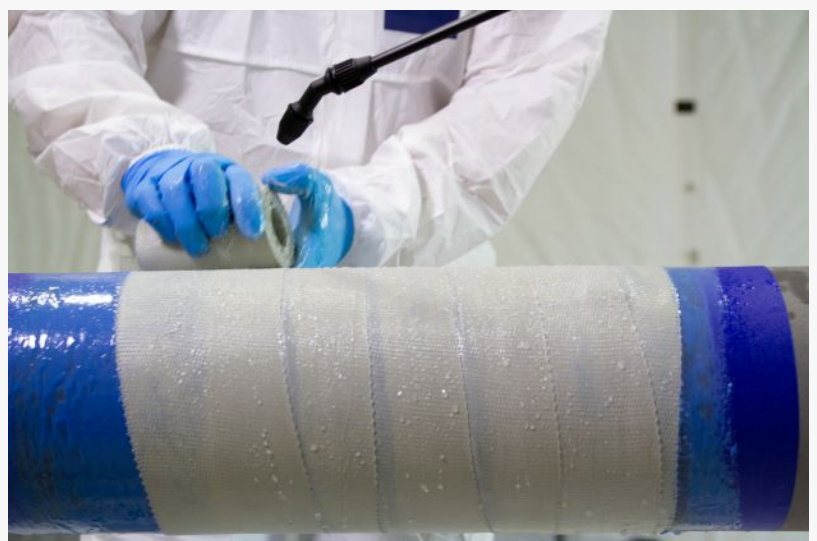
A+ Wrap installation
