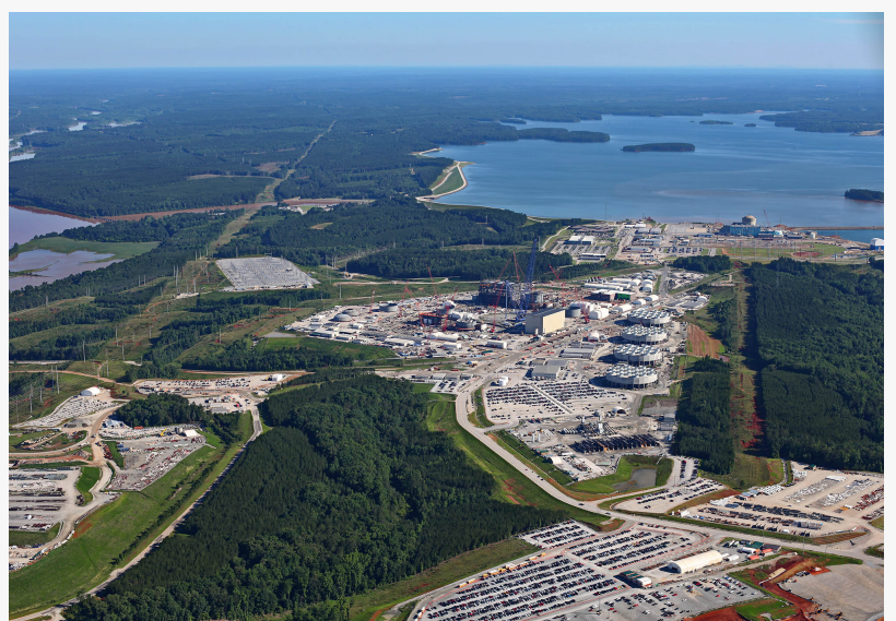
Aerial shot of V.C. Summer site north of Columbia, SC, with two terminated Westinghouse AP1000 reactors in foreground and single operating unit in background; photo ©High Flyer 2017
